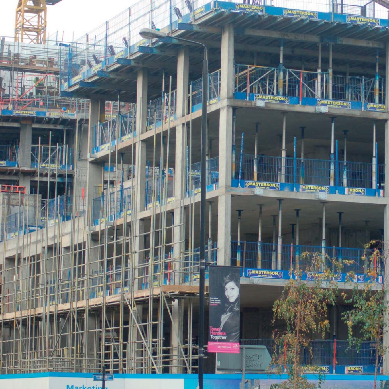
St Andrews under construction
